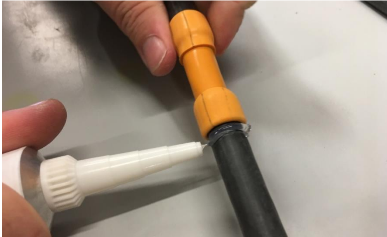
Image 5 : Example of Autoshrink being installed with Glenair Duraelectric adhesive.
