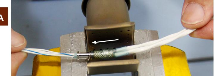
Focus heat on ferrule for a few seconds and begin moving towards the solder preform. Solder should melt and begin to flow freely. Continue to move the preform towards the center of the heat reflector as solder completely melts and flows along preform braid.
