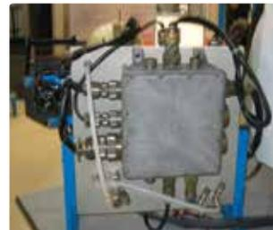
The case was solved with Glenair ITS reverse bayonet connector cables and flange mount receptacles. Plugs with cable clamp backshells mated to receptacles mounted on existing metal junction boxes along with a specially-designed, corrosion-free and EMI/RFI-protected Glenair Composite Junction Box, factory wired to an internal termination block.
