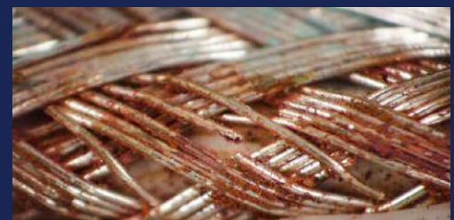
Images of Red Plague corrosion on wire conductor material and braided shielding courtesy NASA.
